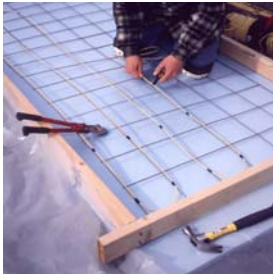
Floorizwarm Heating Element Layout
