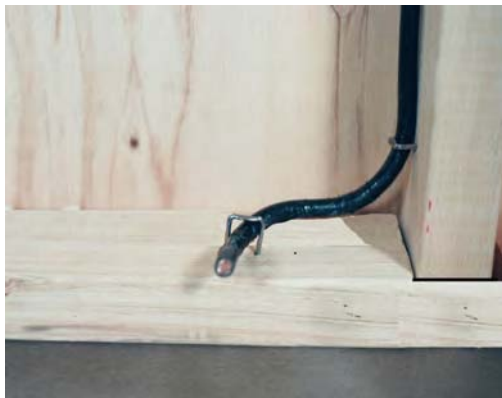
Illustration 1.6 Cold lead roughed-in for wall installation of Transition Plate (E217).
