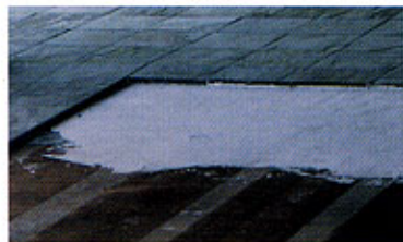
Flooring goes on top of heating material
