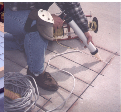
Retrofit Tuff Cable into existing concrete or asphalt or install it in a Heatsink Kit under conductive roofing materials
