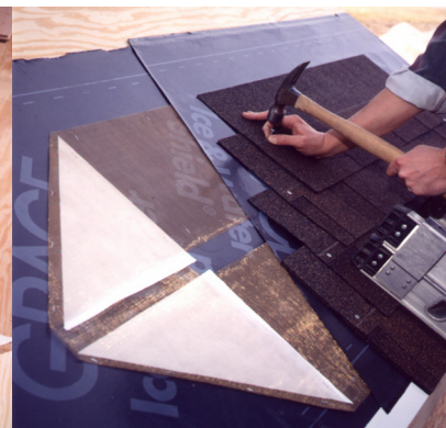
Install Z Mesh under non-conductive roofing materials for safe elimination of snow and ice dams
