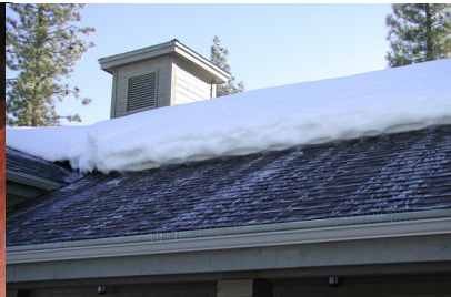
Install Z Mesh under non-conductive roofing materials for safe elimination of snow and ice dams
